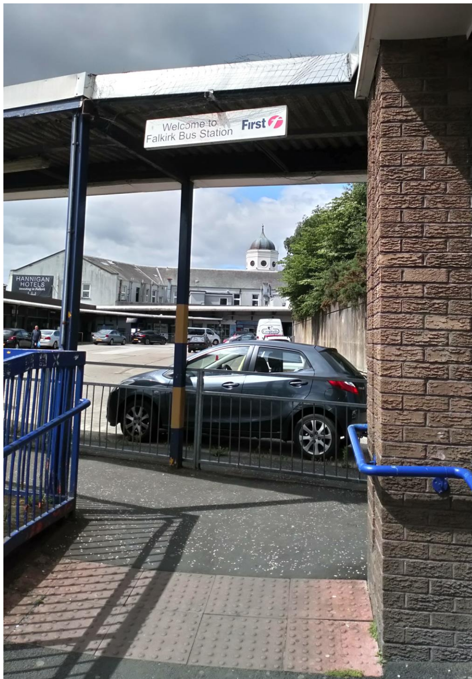
Photo 7 – Falkirk Bus Station after Closure in August 2018 (1)
