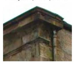
Faulty drainage from this roof is causing damage to the ashlar.
