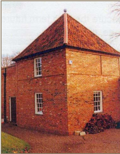
New Pavilions adjoining existing garden wall at Tynninghame House
