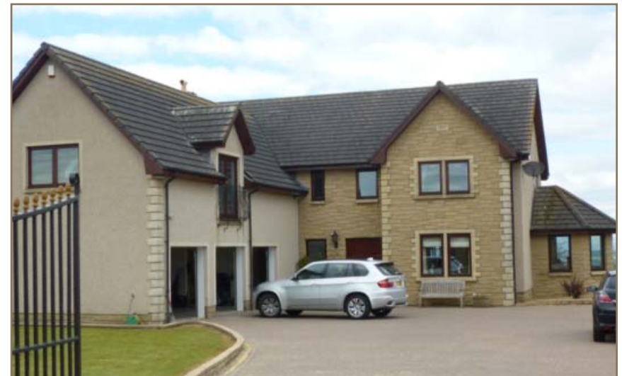
Inappropriate urban architectural style and materials
