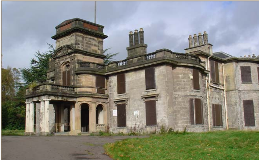
Larbert House : Approved Enabling Development Scheme to support restoration, conversion and extension of Category “B” Listed Mansion
