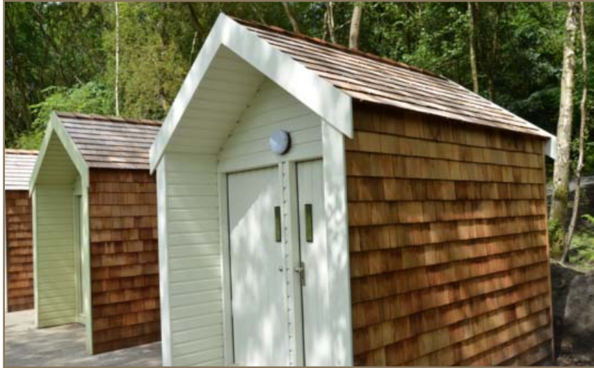
Storage Huts, Causewayend
