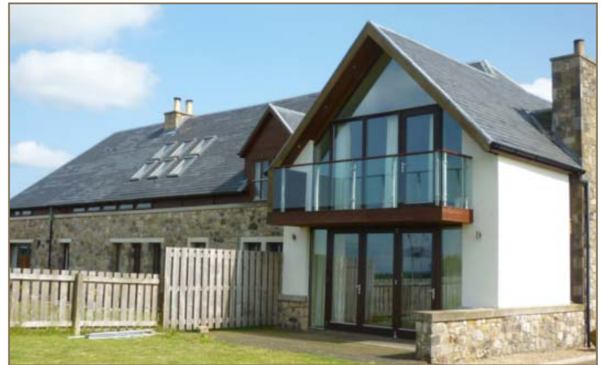
Vernacular buildings can be successfully remodelled and extended to provide contemporary living spaces without sacrificing traditional character
