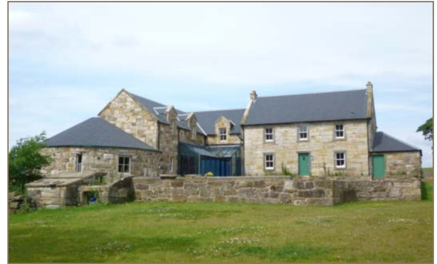
Farm Steading Converted and Extended to Create a Coherent Building Group
