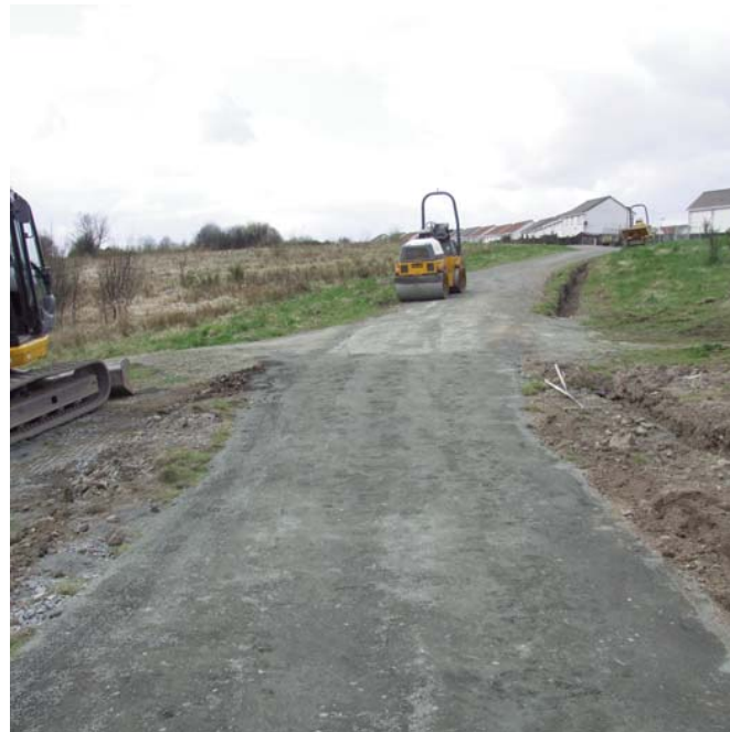
New path link to housing under construction at Bonnyfield Nature Reserve
