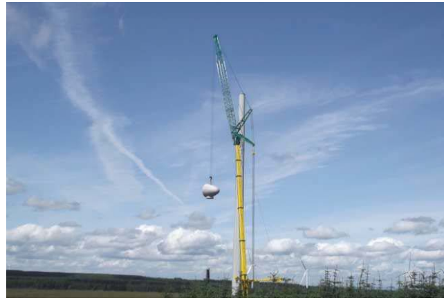
Nacelle lift at WTG19
