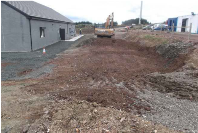
Levelling of car park outside control building
