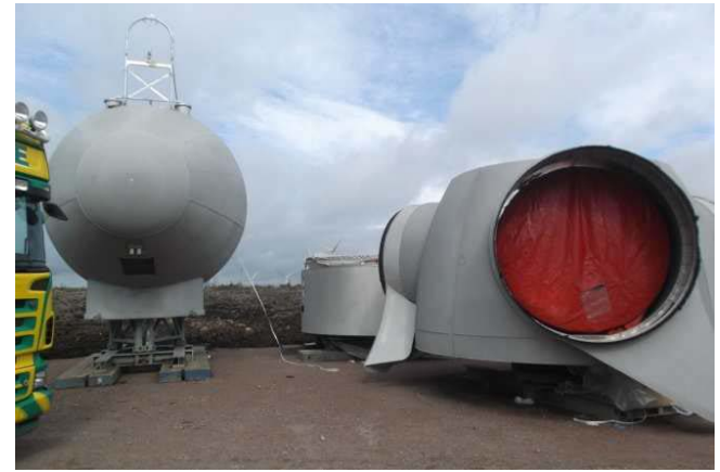
Hub nacelle and generator at WTG9
