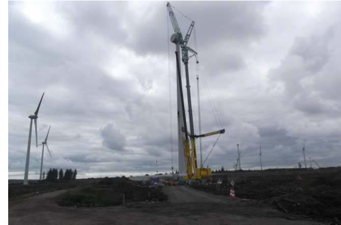
750 tonne crane at WTG 9
