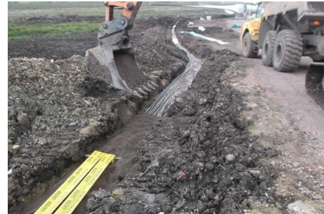
Sand and backfill cables to WTG19
