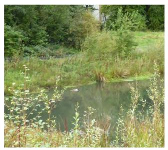
**Mixture:** Developments typically have a SUDS scheme, usually a pond or basin at the bottom of the site. Using a mixture of SUDS such as ponds, swales, green roofs, trees, rainwater gardens etc. throughout the site can help create an attractive and linked green and blue network, mimicking nature and the SUDS management train. Images: Commonwealth Games Athletes' Village, Glasgow
