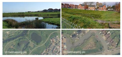
Access for maintenance: Where access to ponds and basins is necessary for maintenance, access tracks should be unobtrusive and integrate with the open space of which they are part, for example through the use of reinforced grass systems. Images: Carrongrove, Stoneywood
