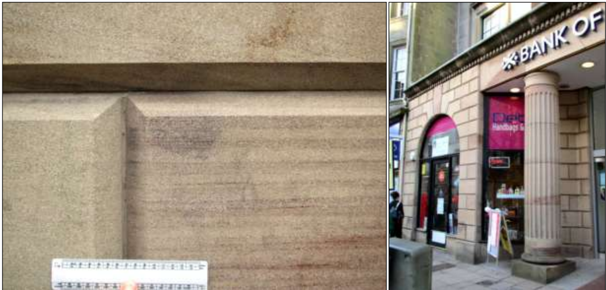
The photograph at right shows the shop front addition to the Bank of Scotland building, which is made entirely of SBM6.
